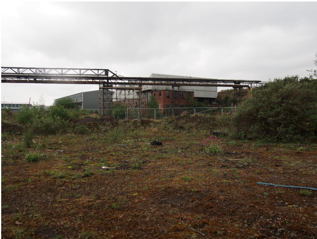
Plate 9: Looking south from the Oxygen plant to the former Loco Shed Repairs shop and Bolckow Industrial Estate beyond.
