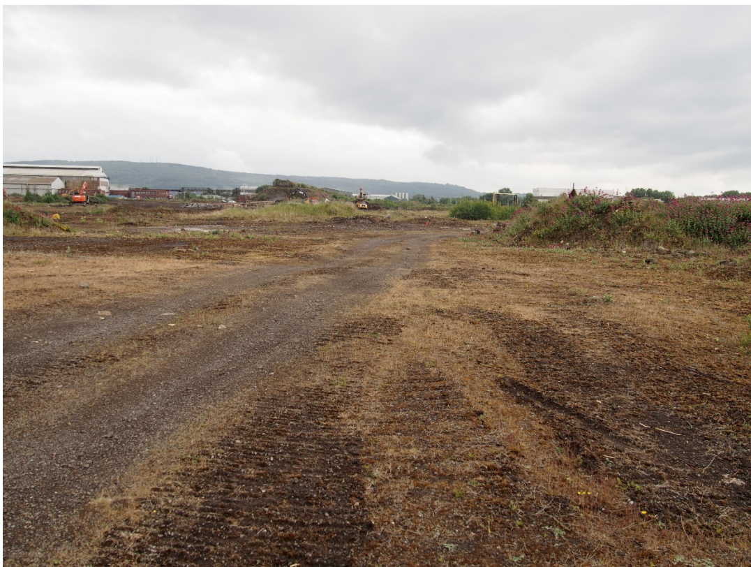
Plate 5: View east towards the Torpedo Ladle Repair Shop
